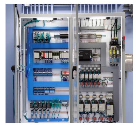
include a UL sticker and verification that all components are UL-Certified. Panels should also have a tag that includes the manufacturer and the project number.
