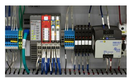
• Components should be arranged in a logical and functional manner. High and low voltage components should be segregated from each other. Since most panels have their main power disconnect switch in the upper right
