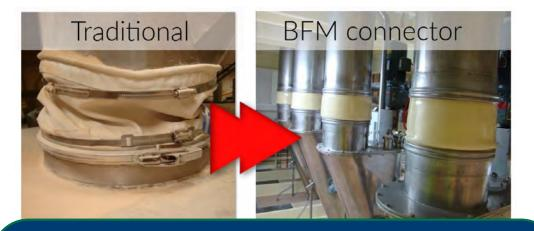
Flexible connectors provide a safe and hygienic alternative to hose clips
